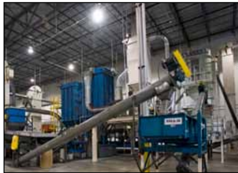
NexTec Group is providing a true end-to-end solution—meeting the challenging requirements of Lehigh Technologies.
